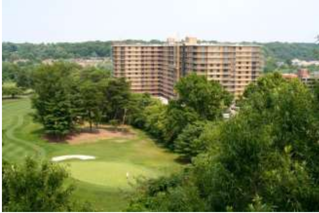
Dolley Madison Towers Overlooking the White #6 Green at Arlington The site of the Dolley Madison Junior High School
