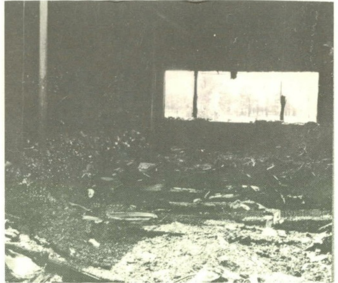
Another view of the Golf Pro Shop fire damage. (photo ANCC)
