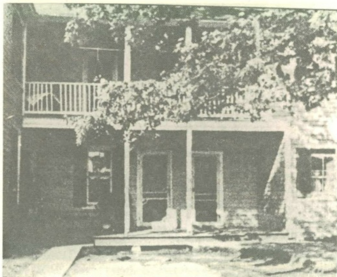
The Swayze House (above) was the original old farmhouse occupying the site of ANCC's Fairfax Club House. (photo No. VA Sun)
