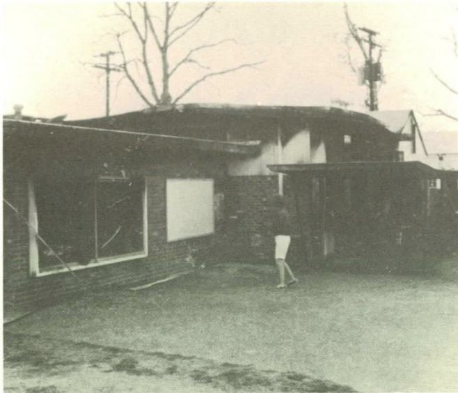
Golf Pro Shop after fire on April 6, 1968. (photo ANCC)
