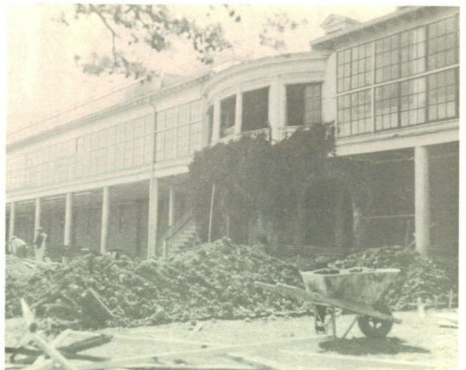
Demolition preparatory to sun room/grill extension March 14, 1939. (photo ANCC)
